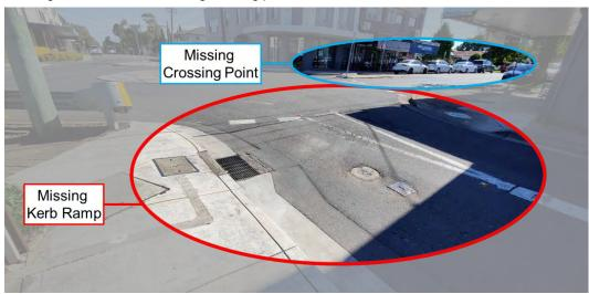
Figure 8.4: Missing Crossing Points at the Northern and Eastern Legs of the Intersection Redundant Footpath
