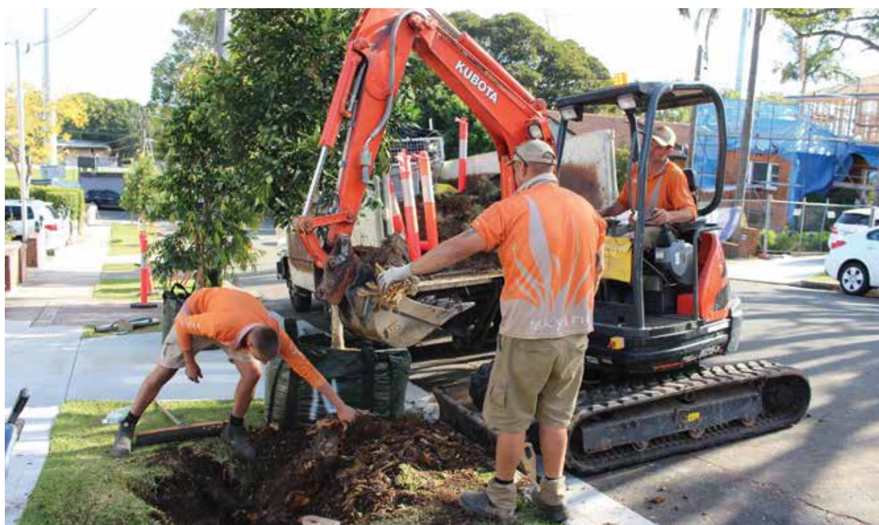
Photo: Council is steadily replacing problem trees and repairing footpaths to ensure the safety of the community.
