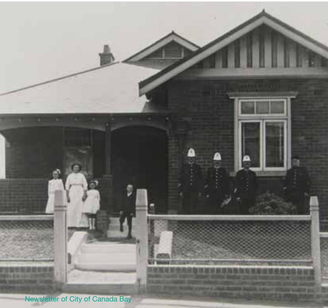
The old Five Dock police station on the site of what is now Fred Kelly Place
