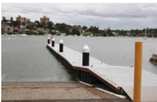
The jetty, carpark and boatramp at Taplin Park has been upgraded, providing improved access for water users.
