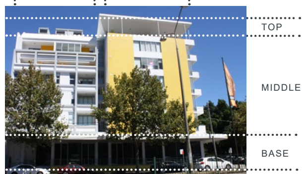
Example of a building that is vertically articulated into two components and differentiates between base, middle and top
