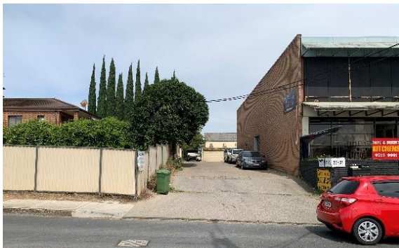
Figure 4.4 Boundary between the rear of Courland Street lots (Kings Bay East) and State Significant Development (SSD) site to the west, prior to demolition of SSD site.
