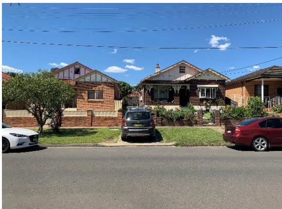
Figure 4.8 Taylor Street, east side.
