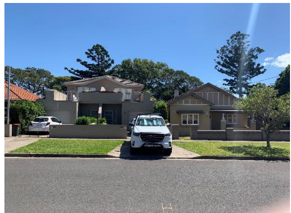
Figure 4.9 Taylor Street, west side.
