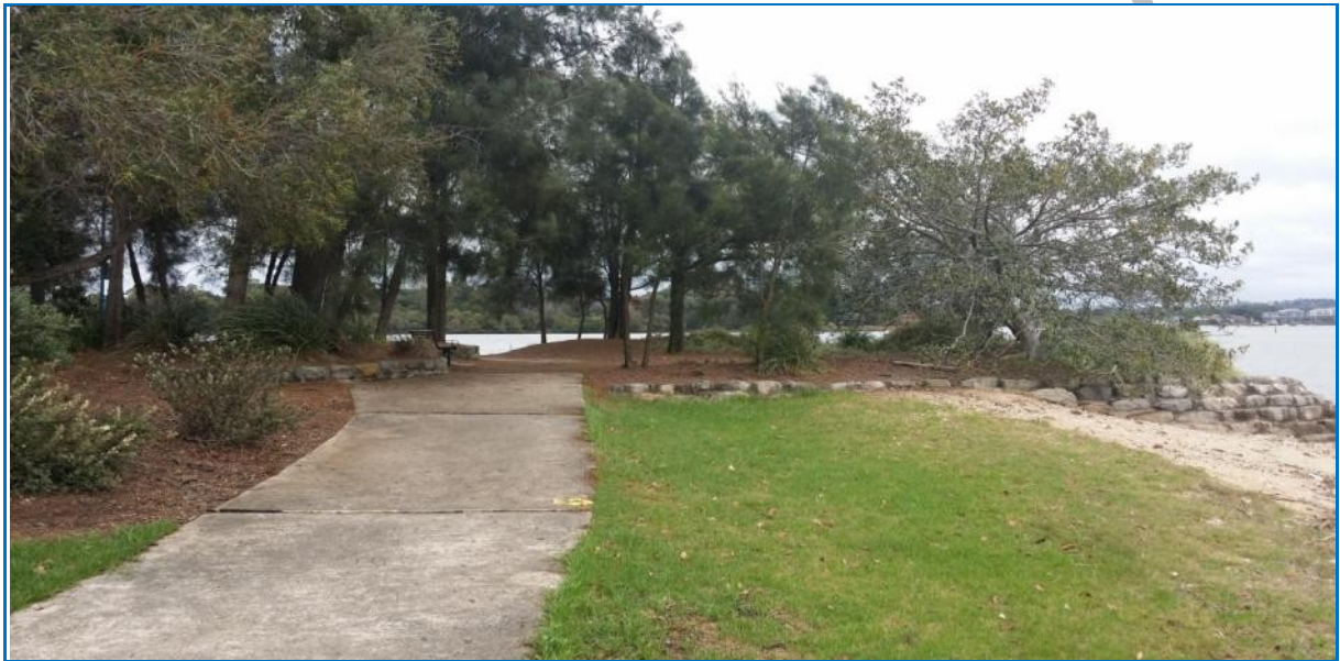
Figure 4.4: The existing concrete path and broader concrete apron around the point is in disrepair. In this locality, it is likely to seal fill used to raise the Point above current high tide levels
