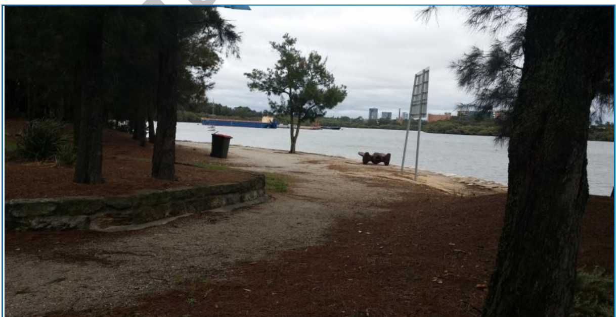
Figure 4.4: The existing concrete path and broader concrete apron around the point is in disrepair. In this locality, it is likely to seal fill used to raise the Point above current high tide levels
