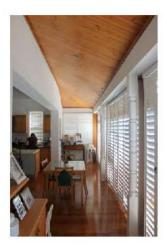
Figure 3.15 3 Wolseley Street, Drummoyne Infilled verandah – the columns are later replacements
