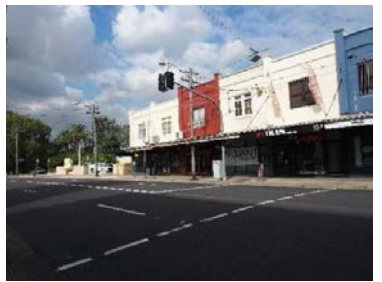
Figure 9 View of 1 and 7 Ramsay Road The subject site has a prominent frontage which has the potential to provide an active ground floor to revitalise the neighbourhood centre character. Source: Architectus (2018)
