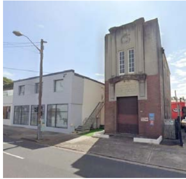
Figure 11 View of Electricity Sub-Station located north east of 1 Ramsay Road. The height of the electricity substation matches the height outcome of the control.
