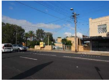
Figure 7 View from the intersection of 1 and 7 Ramsay Road and Henley Marine Drive. Photograph identifies the previous Roads and Maritime Services building currently occupying 1 Ramsay Road. Source: Architectus (2018)
