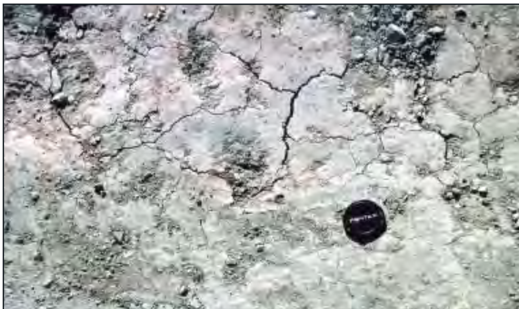
Figure A4 Smooth and compact ground surface typical of an urban construction site, raising the P-factor as high as 1.3
