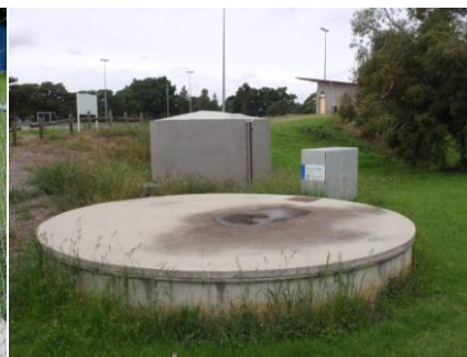
Stormwater harvesting tank
