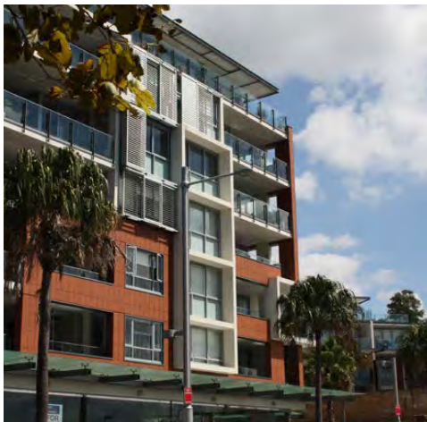
Example of balconies with a balance of solid and void in the facade composition and treatment.
