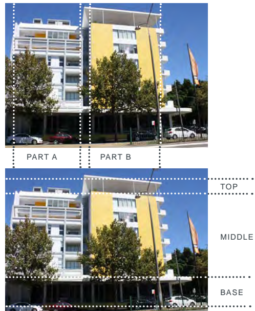
Example of an building that is vertically articulated into two components and differentiates between base, middle and top
