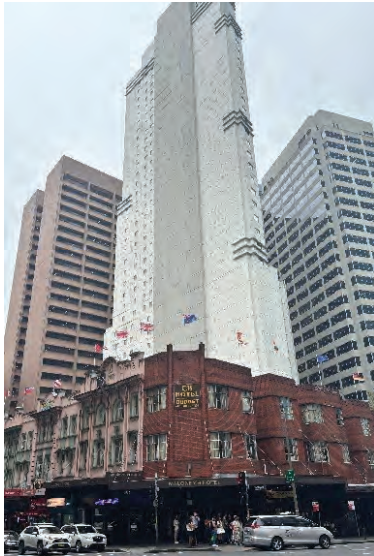
Figure 2, Blank facade to an approximately 35 storey building, Cunningham St, Haymarket
