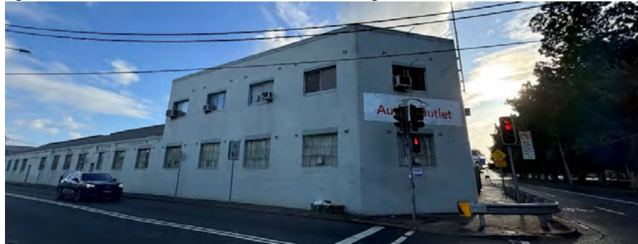
Figure 4 View of the Develotek site from the corner of Queens Road and Williams Street (looking south-west)
