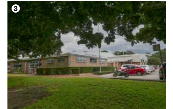
3 Five Dock Leisure Centre
