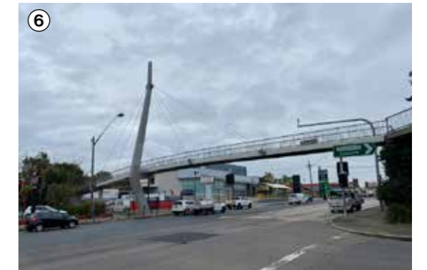
Pedestrian bridge on Parramatta Road
