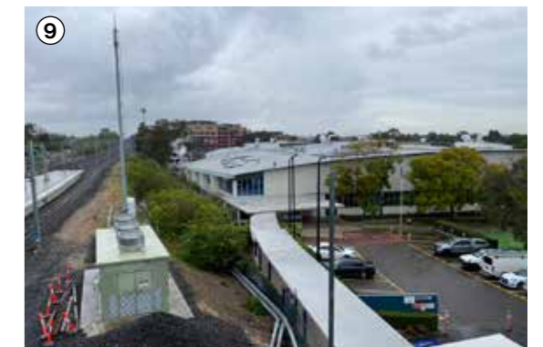
Industrial building next to the train station
